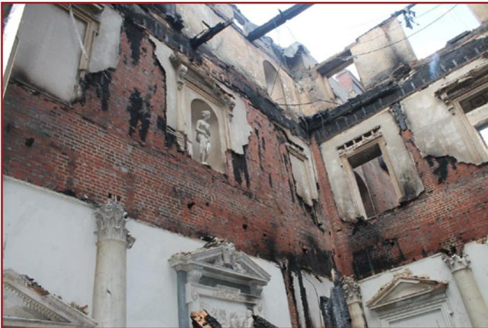
After effects of a fire believed to have spread through open voids having originated in a basement plantroom
