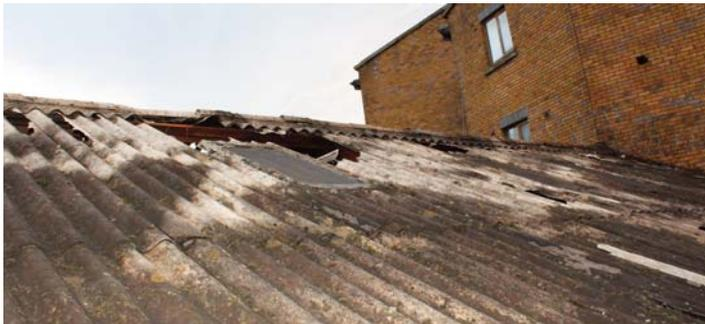
Asbestos Cement Roof Sheets damaged by Fire
