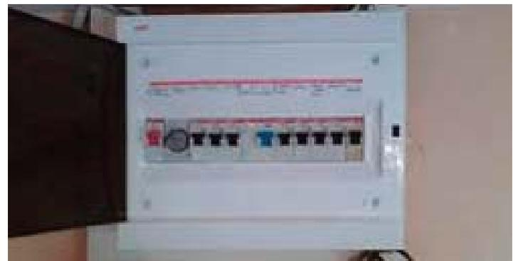
Electrical indicators – operation of MCBs can provide information on the circuits which were first affected by fire or where incident appliances were connected.
