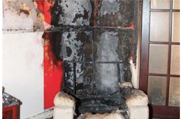
Geometrical patterns – patterns of burning that have resulted on various surfaces; floor, walls, ceilings. Areas of clean burn (no soot) are interesting as the temperature has been high enough to burn off the carbon and soot depositing on this area. Smoke venting from openings and collapse of structural members including roofs and walls should be noted.
