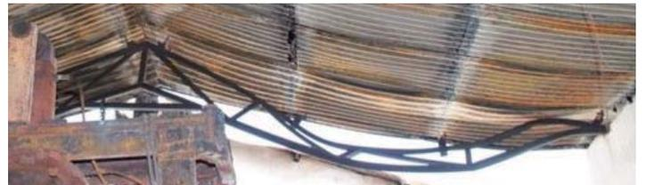
Time/temperature patterns – depth of char, spalling of concrete, calcination, distortion of steelwork.
